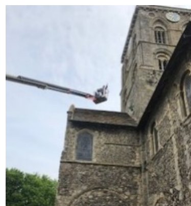
Inspection of tower stonework
